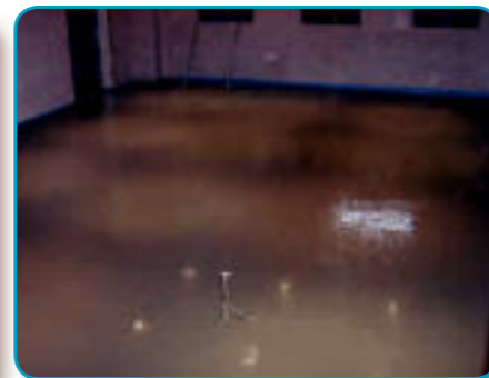
■ e screed should be laid whilst the pipe is pressurised.
